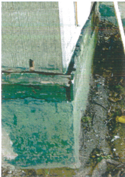
Example of a Rotten Sill Plate
