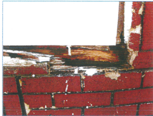
Example of Deteriorated Window Framing
