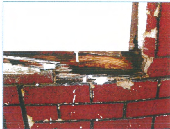
Example of Deteriorated Window Framing
