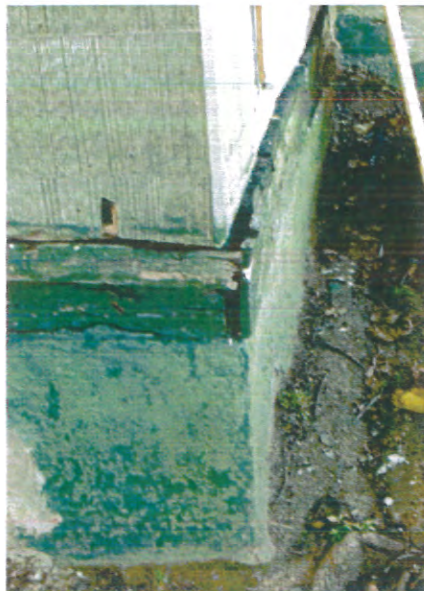
Example of a Rotten Sill Plate
