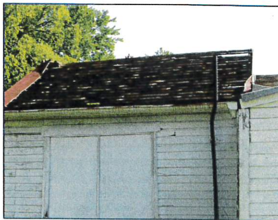
The Metal Roofing Was Stripped from this House to Sell to a Scrap Dealer
