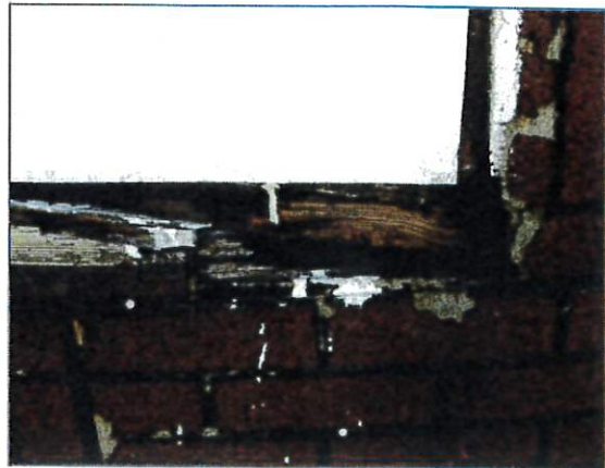
Example of Deteriorated Window Framing
