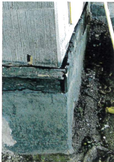
Example of a Rotten Sill Plate
