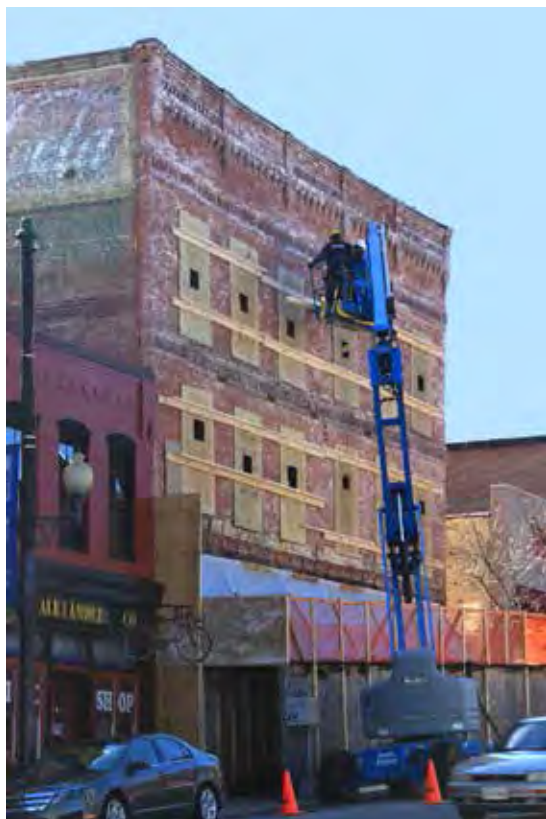
The Ferrell Building on Main Street during restoration (left), and right after completion in 2012. Among the problems to be solved was a buckling of the facade which threatened the entire building. Restoration by Rehab Builders of Winston-Salem, with financial assistance from the City.
