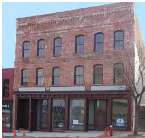
The Ferrell Building on Main Street during restoration (left), and right after completion in 2012. Among the problems to be solved was a buckling of the facade which threatened the entire building. Restoration by Rehab Builders of Winston-Salem, with financial assistance from the City.
