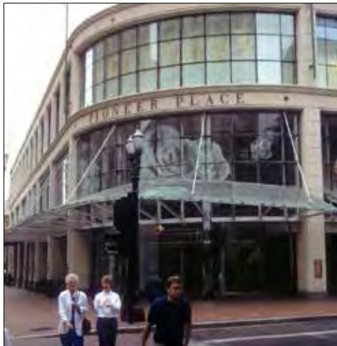
Modern clear canopy supported by metal structure.
