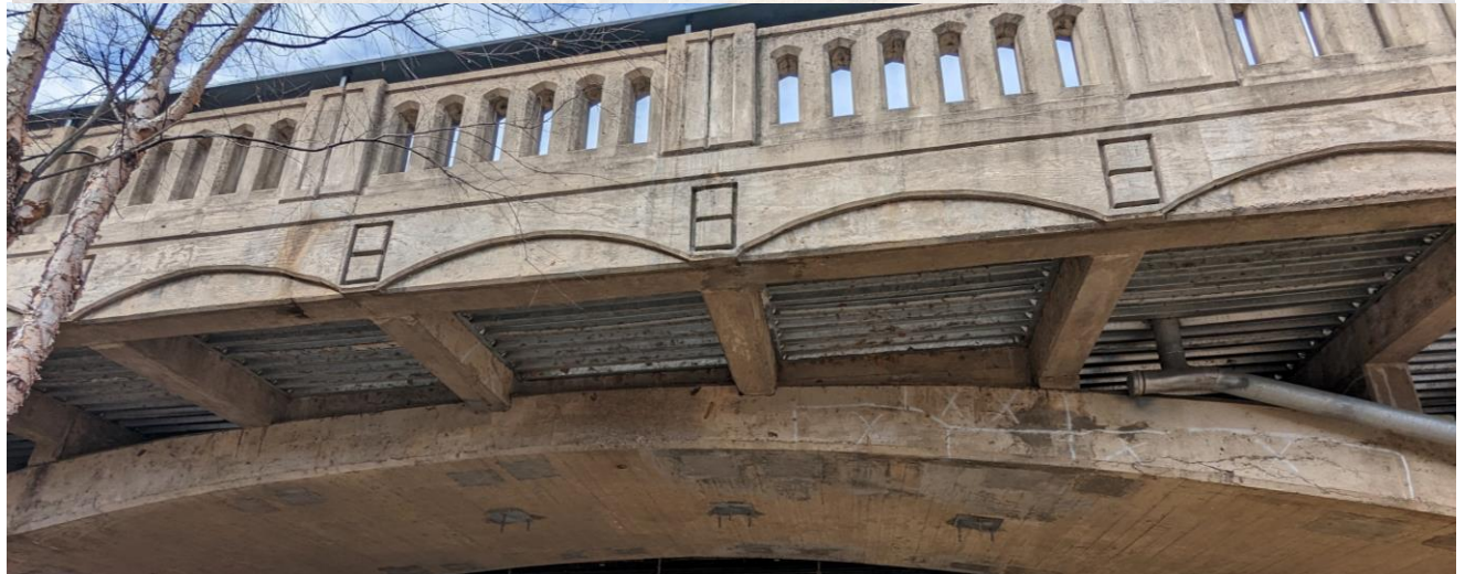
Close up of Original Arch Remaining and newer bridge element above the arch
