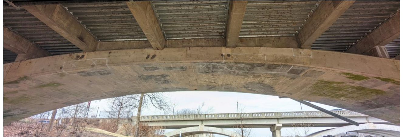
Close up of Original Arch Remaining and newer bridge element above the arch
